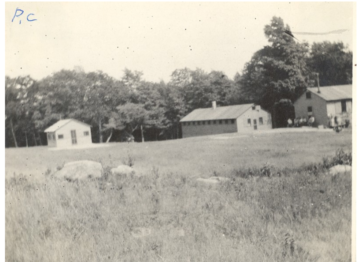
Several buildings were constructed for the fifty prisoners living in the prison camp.
